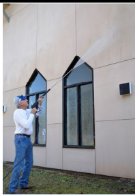
Ricky Howes cleans the exterior walls.
